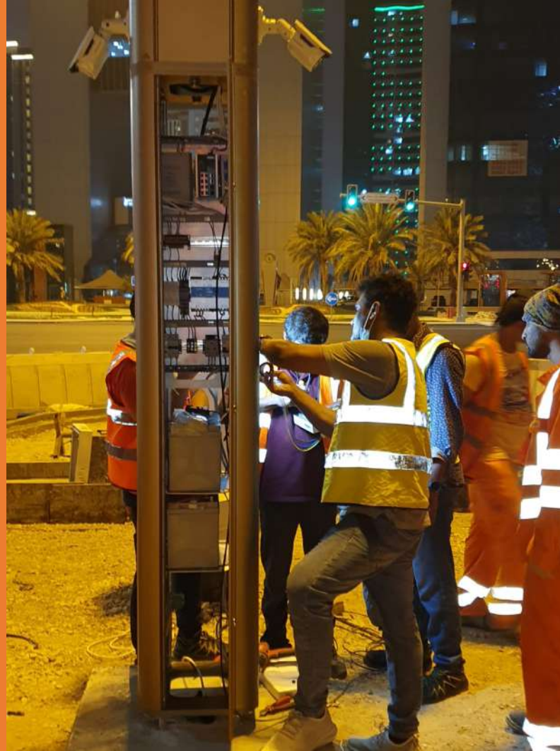
Double door access to twin batteries bank and MOI Surveillance. Doors are integrated into pole without hinges and each door has two security locks. Pole Location City Centre West Bay.
