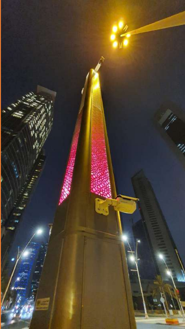
Double door access to twin batteries bank and MOI Surveillance. Doors are integrated into pole without hinges and each door has two security locks. Pole Location City Centre West Bay.
